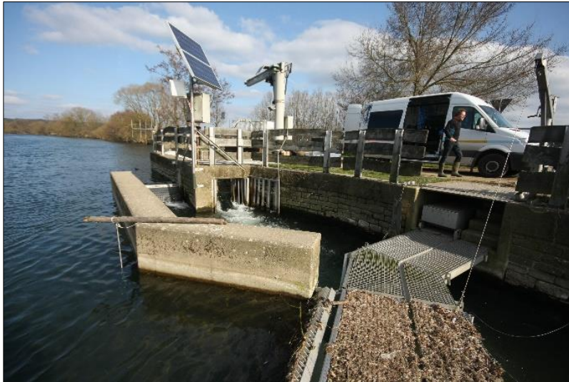
Figure 2.6. Details from the Buisdorf dam.
