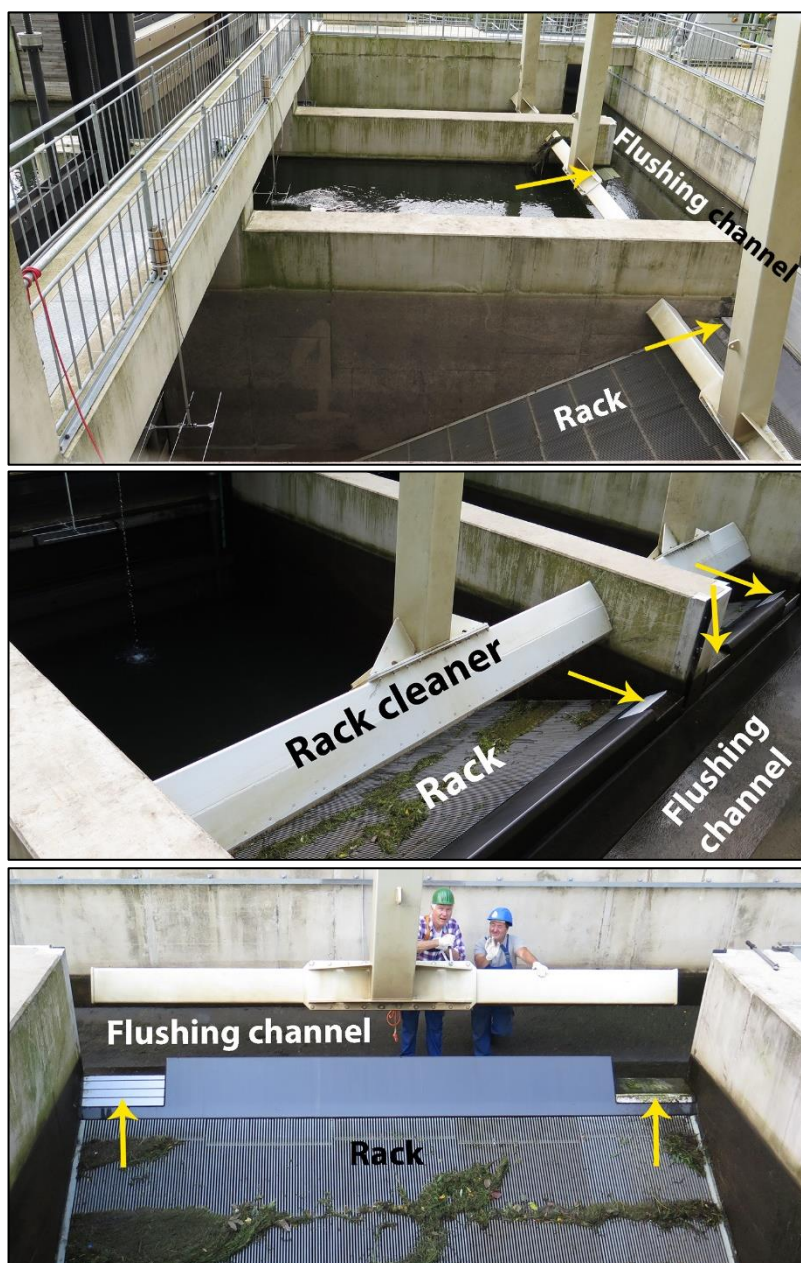
Figure 2.3. Details from the turbine intake at the Unkelmühle power station.
