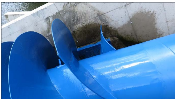
Figure 6.2. The upper part of the Archimedes screw turbine at Kuhlemühle in the Diemel. Photo by Eva B. Thorstad.
