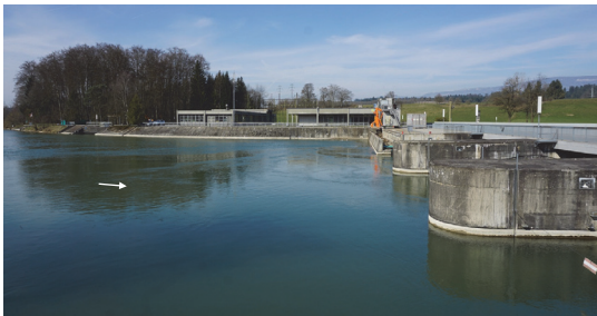
Fig. 1: Head water of block-unit HPP Bannwil with the turbine intakes in the background (Photo: VAW)
